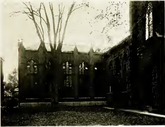
Addition to Osterhout Library (Stack Room) South Franklin Street
